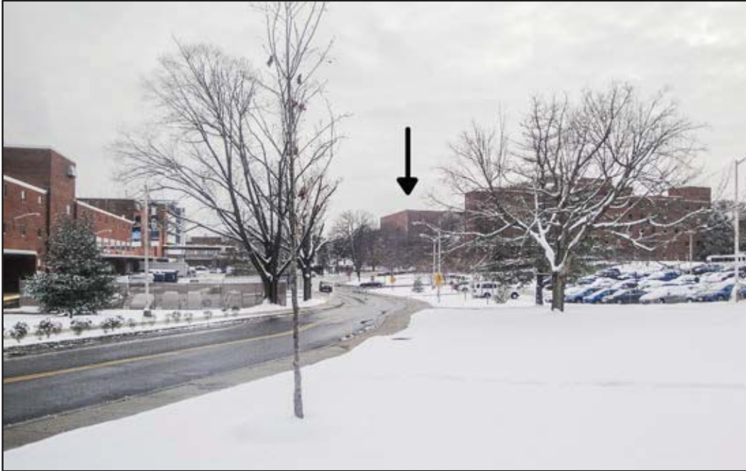
Figure 3-15. View of Building 34 from Central Campus (near Building 10)
