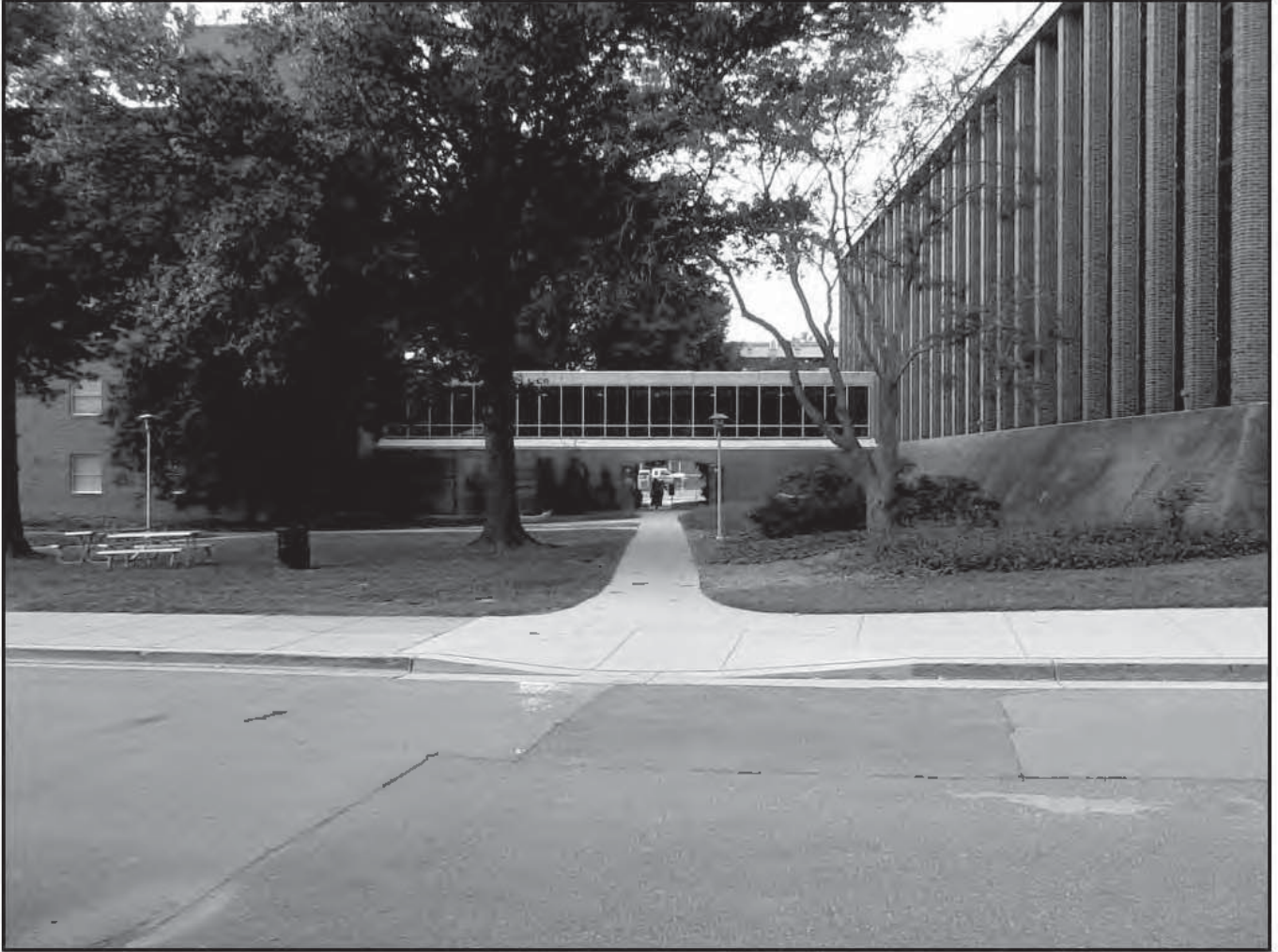
Photo 4: View of North Elevation of Connector Bridge Between Buildings 29 and 29A, 2012
