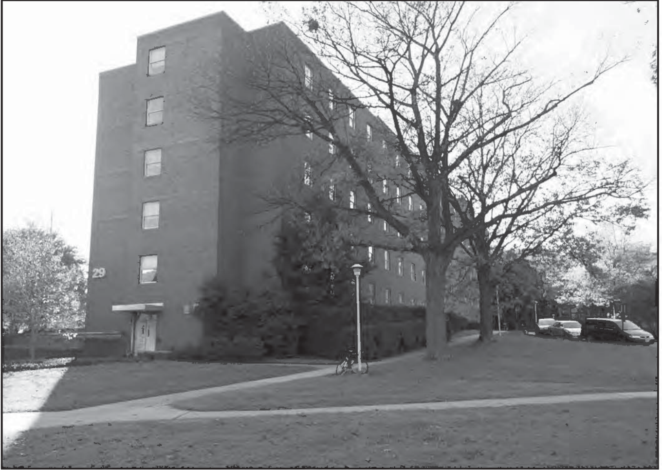
Photo 2: Oblique View of the Northeast Corner of Building 29
