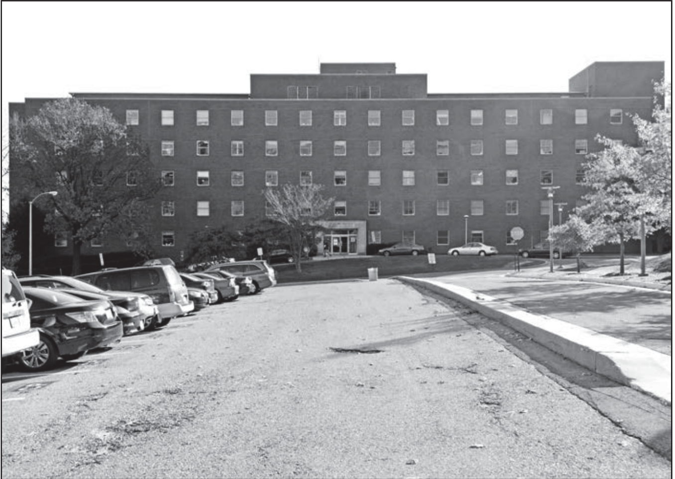
Photo 1: View of the Main (North) Elevation of Building 29
