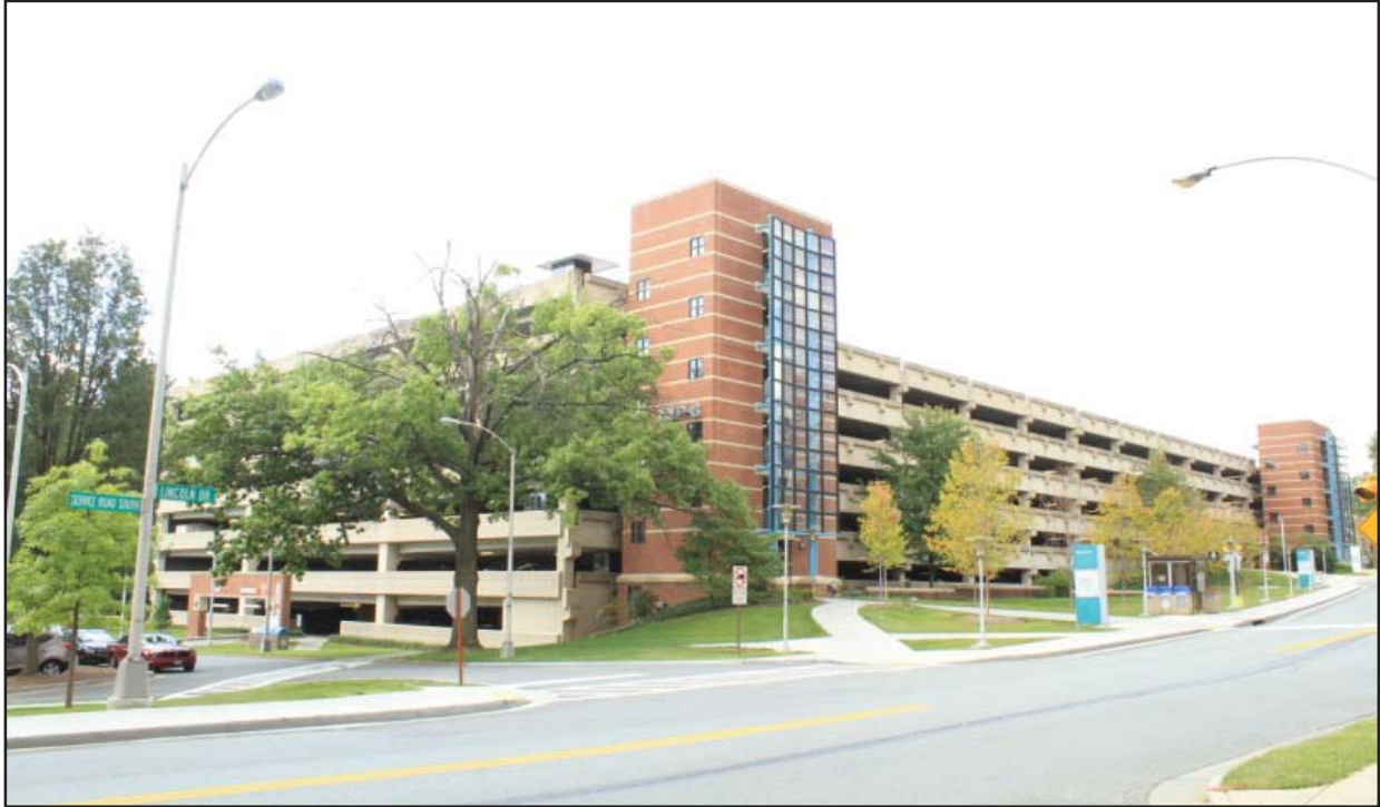
Figure 1-4. Example of Existing Parking Garage (MLP-8) on Campus
