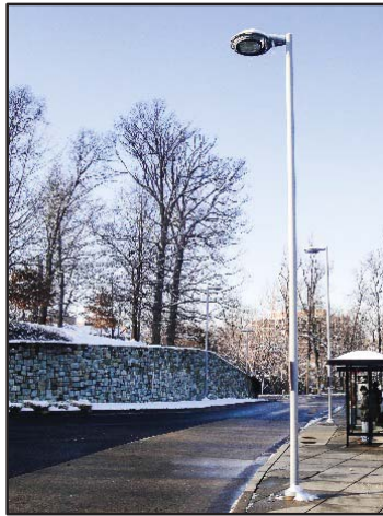
Figure 3-11. Example of Newer Streetlight Fixture
