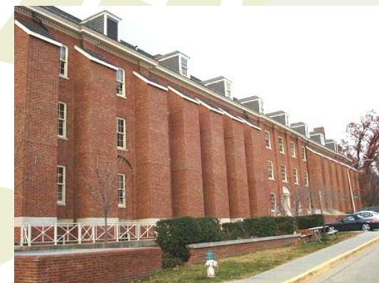
Building 4 (1st and 2nd floors will be certified Silver)
