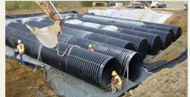
Once completed, these underground detention pipes will aid in slowing down runoff water from the NIH's Clinical Research Center before it reaches the NIH stream.
