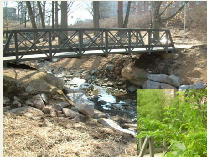
(Above/ Right) Before and after photos of the stream restoration project. The above photo is from 2004 and the photo to the right is from 2006.
